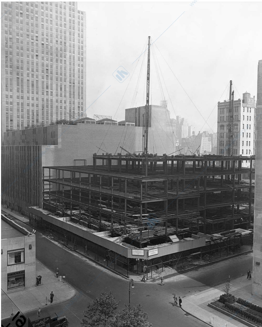
[46] Cantiere Rockefeller Center 1930
